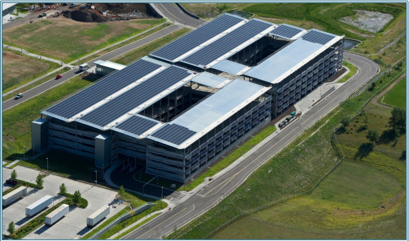
A parking garage at the National Renewable Energy Laboratory, with much of the roof space covered by solar panels. Government agencies can lead by example to demonstrate the feasibility of renewable energy installations, as well as energy efficiency and conservation practices (NREL 2012b).
