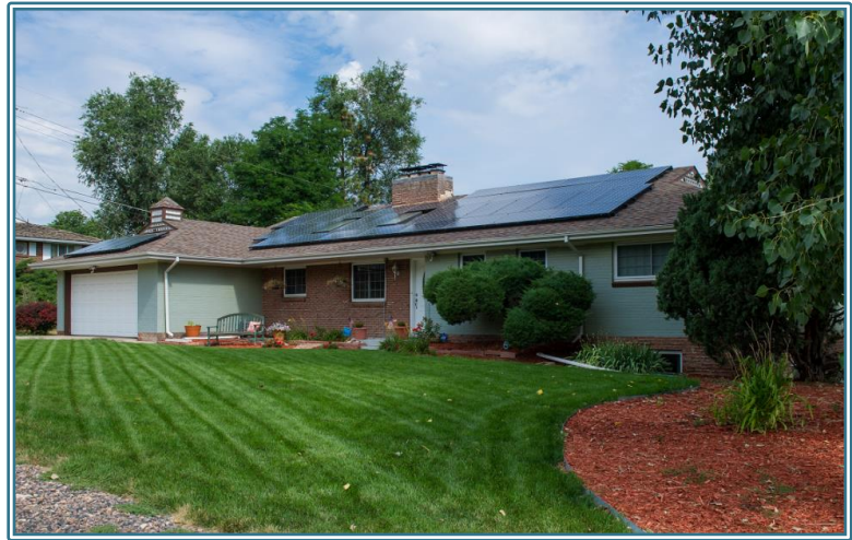
Renewable energy technologies can be installed in large fields of hundreds or thousands of acres. Alternatively, they can be used in small-scale installations, such as the photovoltaic panels on the roof of this home (NREL 2014).
