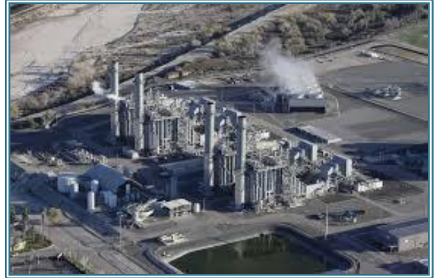
Southern California Edison's Mountainview Generating Station in San Bernardino County is one of the most efficient in the state. Although natural gas burns much cleaner than some fuels such as coal, this plant is one of the largest contributors of greenhouse gas emissions (CO 2 ) in the state according to the Environment California Research & Policy Center.
