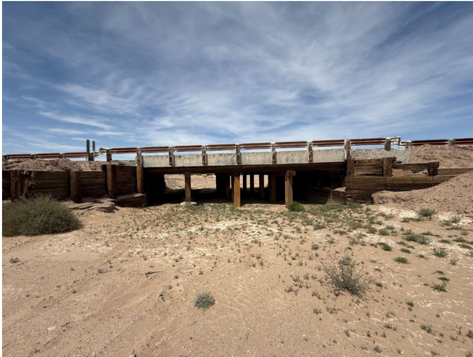
Representative Photo 1. Lamego Ditch bridge, facing north.
