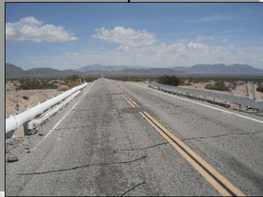
Photo 1 - Ground View of Bridge
