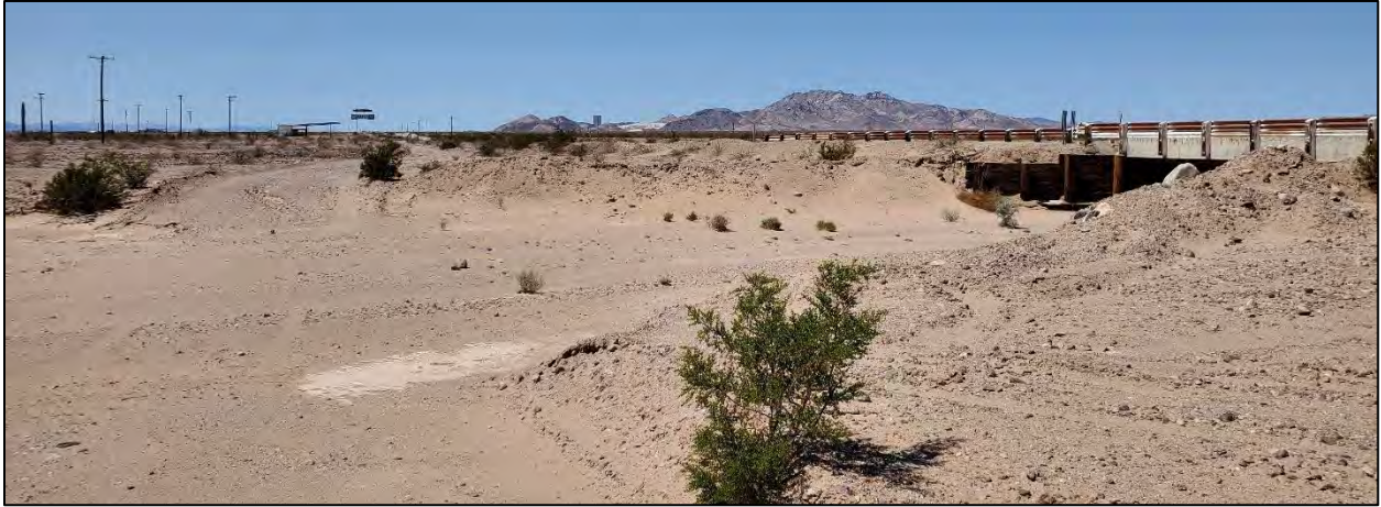
Figure 6. Lamego Ditch Bridge overview
