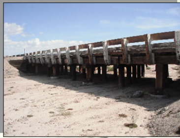
Photo 2 - Ground View of Bridge
