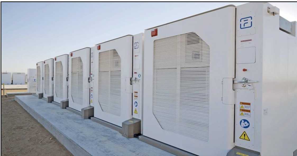
Figure 10 - BESS ENCLOSURES
