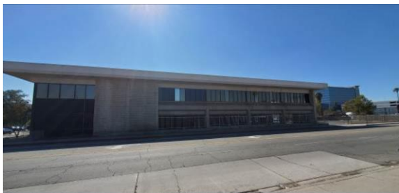
Figure 2-3: North Building Elevation
