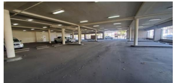
Figure 2-7: Parking Level (Westward)
