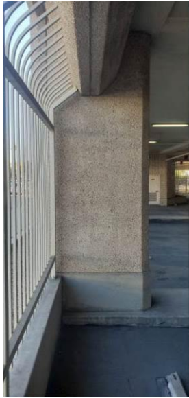
Figure 2-9: First Level Concrete Pier
