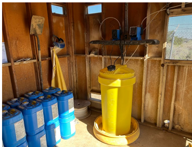
Chlorine Dosing for Wells 1 and 2
