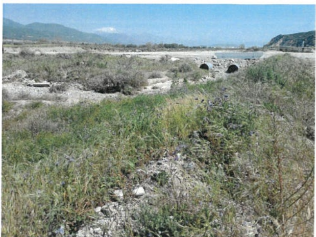
Photo 16: View looking south at an existing drainage that flows underneath Glen Helen Parkway, and spills out onto floodplain of Cajon Wash.
