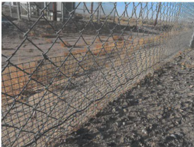
Figure 3 Existing Tortoise Fencing
