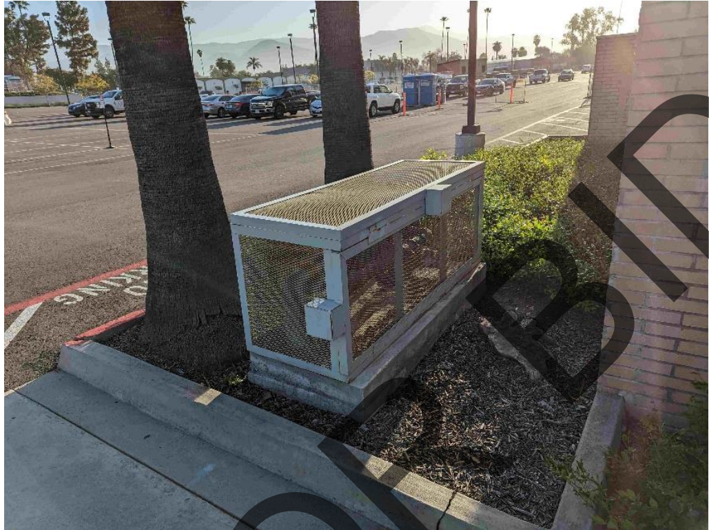
Detail 2/EXT – Water Backflow Preventer
