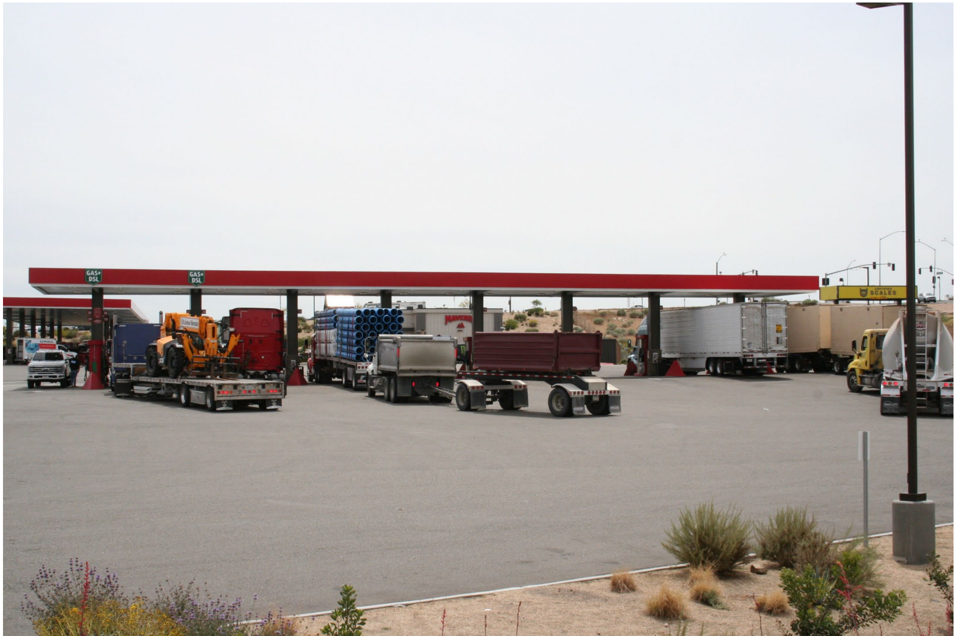
Regional diesel truck fueling facility
