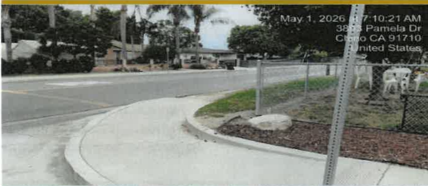
Photo 6. Curb return on Pamela Dr near the school driveway — no ADA ramp serves this corner.
