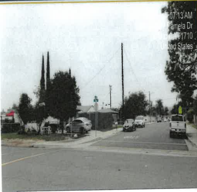
Photo 14. Cozzens Ave / Pamela Dr intersection — no high-visibility crosswalk markings on either leg.
