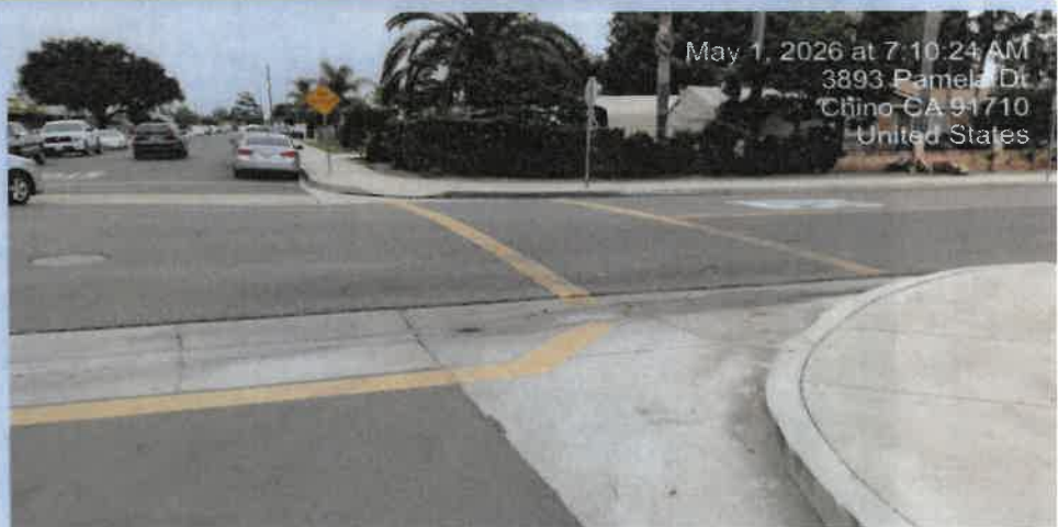
Photo 2. Curb return at the school entrance — no truncated dome warnings or ADA-compliant ramp at this corner.
