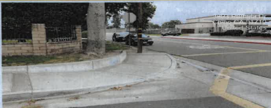
Photo 3. Faded standard crosswalk striping at the school crossing — no high-visibility (continental) markings.
