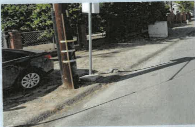
Photo 11. Roswell Ave (Google Street View) — utility pole sits in the planned walkway alignment; vehicles park on bare dirt where the sidewalk should be.
