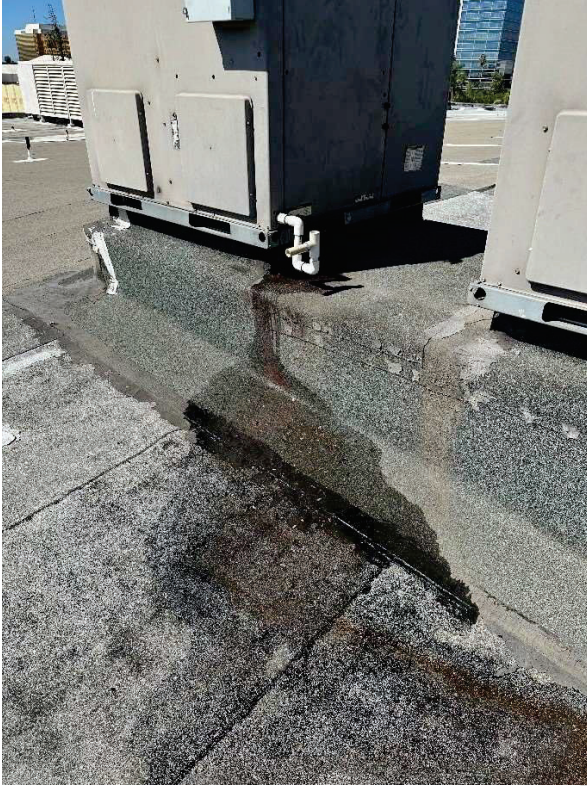
M7 – typical heat pumps leaking condensate
