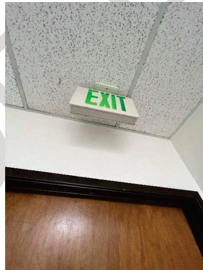
E23 - Typical exit illuminated signage along egress path
