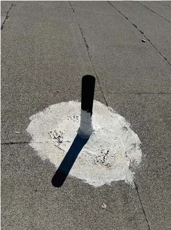
P3 – typical existing plastic roof vent
