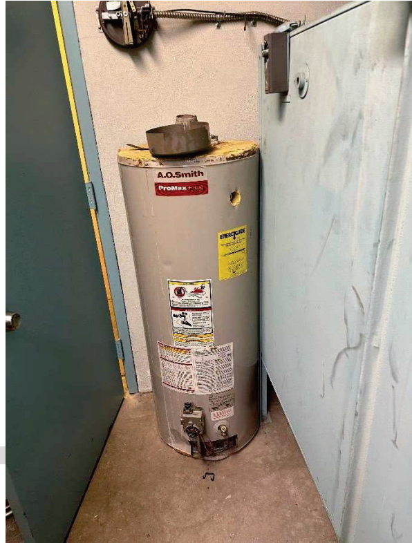
P6 – abandoned water heater in mechanical room
