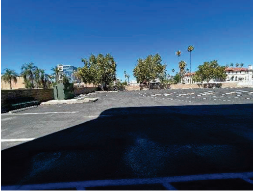
E1 - SCE Utility Transformer 500KVA, 12KU - 480/277V #P5055246 with 8' x 10' Slab box @ Parking Lot
