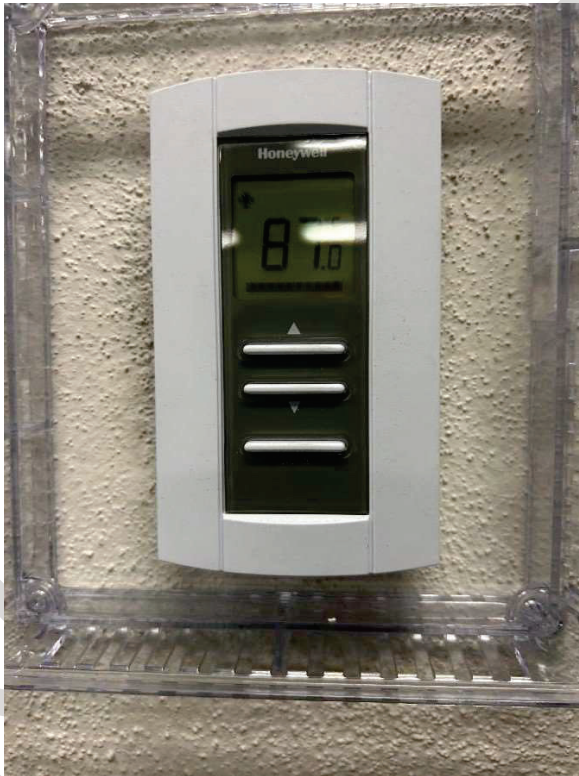
M17 – typical vav box thermostat
