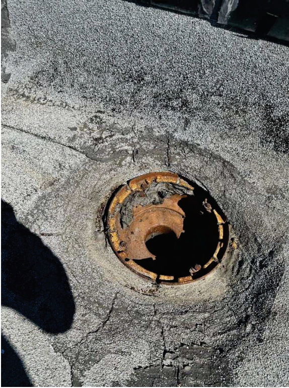
P1 - roof drain without cover
