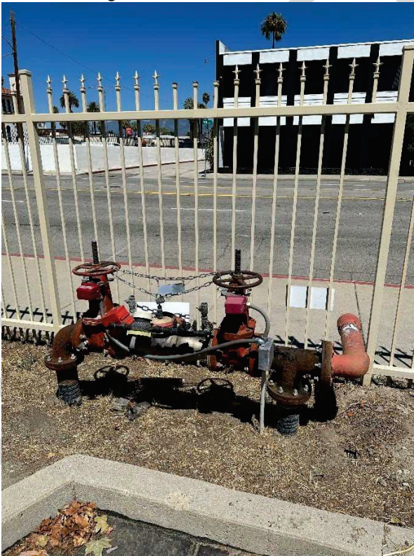
P23 – existing fire sprinkler backflow preventer
