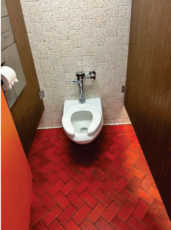
P17 - typical existing flush-valve water closet
