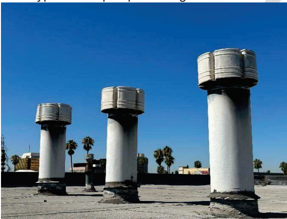
M9 – existing duct furnace flue
