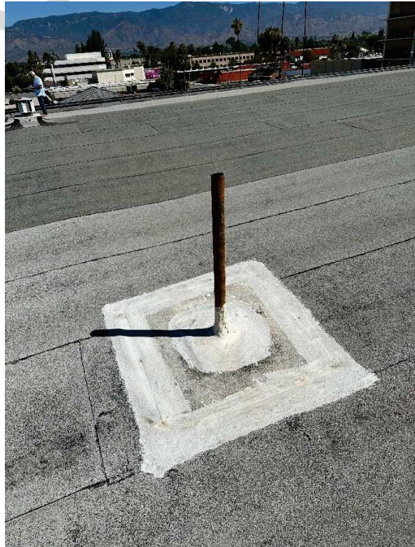
P4 – existing metal roof vent
