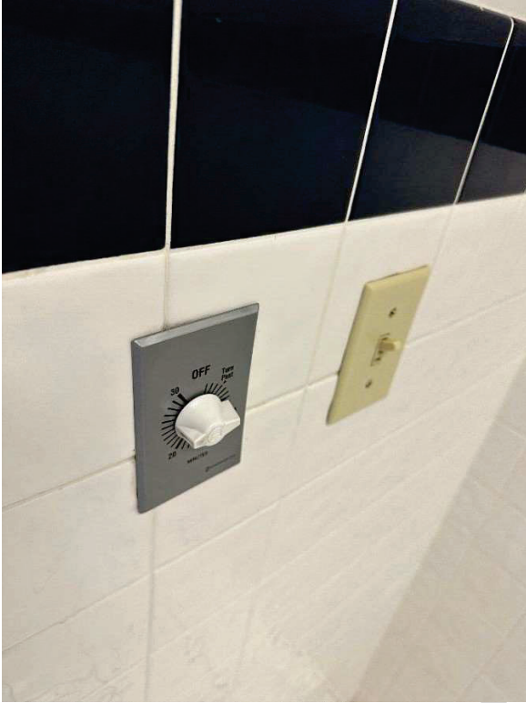
P9 – typical existing time clock exhaust fan in private rest room
