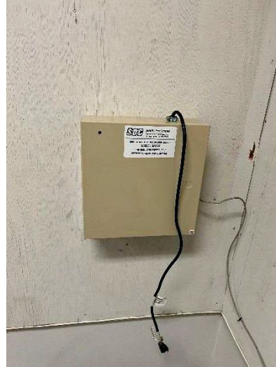
E31 - Security Door Control Cabinet in 2 nd Floor Telecomm Room
