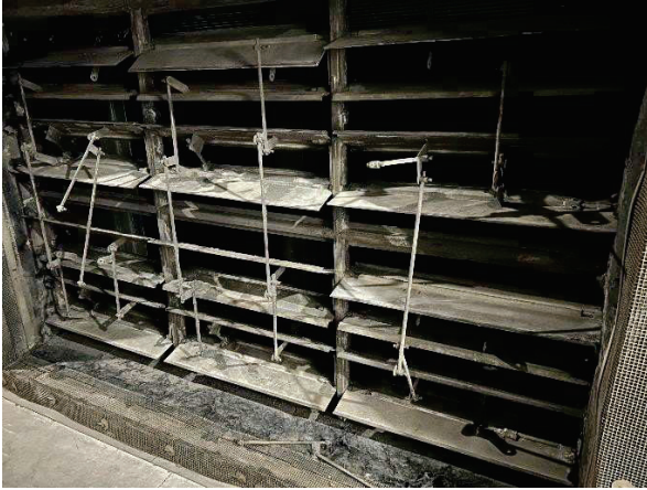
M11 – existing damper linkage
