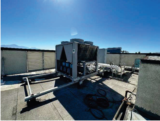
M1 – existing air – cooled chiller
