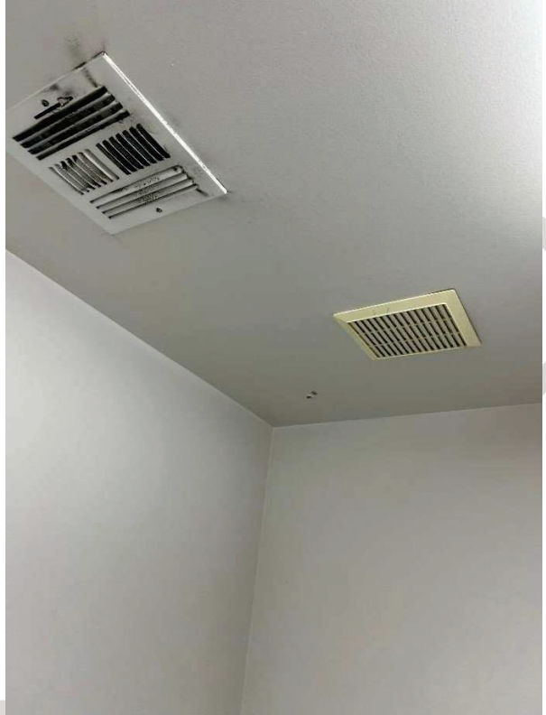
M20 – typical surface mount type grill
