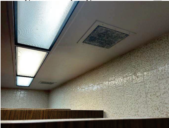
M21 – typical surface mount diffuser
