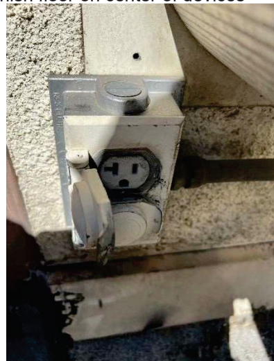
E11 - Typical communications and power receptacle outlets with mounting heights of 16" above finish floor on center of devices
