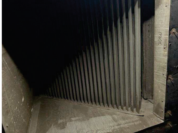
M12 – existing fresh air intake
