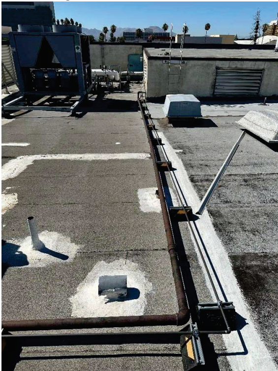
M3 – roof gas piping without roof support
