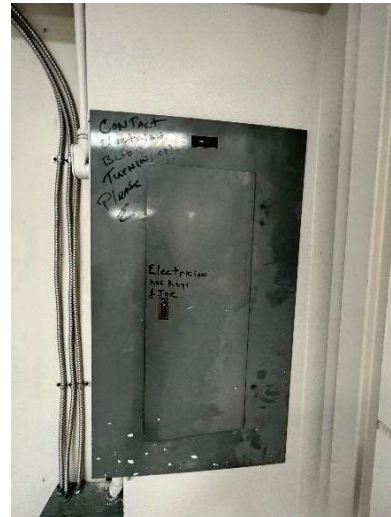
E6 - Panel LA 3P225A, 120/208V, 3P, 4W @ 2 nd Floor Stair Closet
