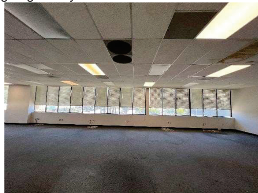
E19 - Typical 2' x 4' recessed fluorescent fixtures at offices
