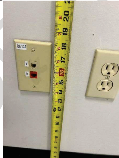
E11 - Typical communications and power receptacle outlets with mounting heights of 16" above finish floor on center of devices
