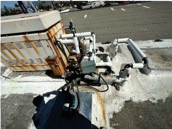
M5 – existing hot water boiler piping assembly
