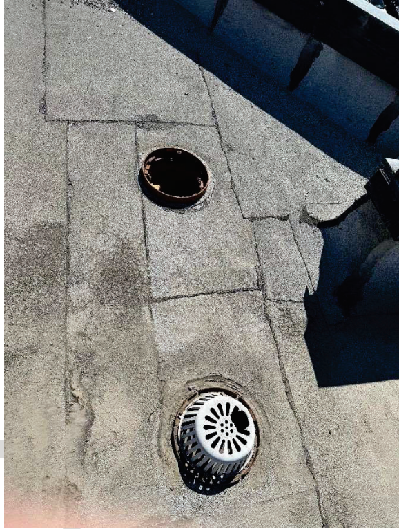
P2 – damaged roof drain cover
