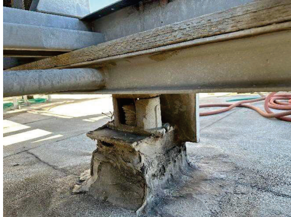
M2 – existing air-cooled chiller roof curb mount
