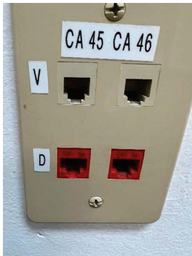
E32 - Typical voice/data jacks utilizing CAT5E horizontal cabling
