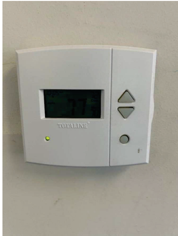
M16 – typical heat pump thermostat
