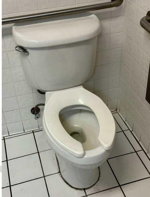
P10 – typical existing flush-tank type water closet in private restroom
