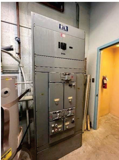
E3 - MCC 3P600A, 3P, 3W 480V (1981) @ 2 nd Floor Mezzanine
