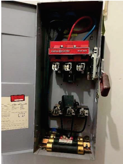
E14 - Typical elevator equipment disconnect switch without auxiliary contacts for proposed elevator recall function (1981))
