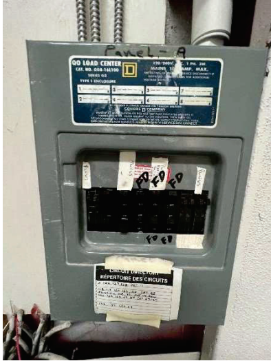
E7 - Panel A 2P100A, 120/208V (1981) @ 2nd Floor Stair Closet
