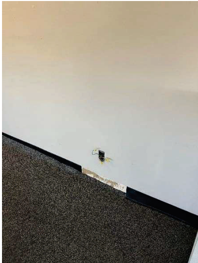
E10 - Open power outlet box without devices @ 2nd Floor Clerical Office
