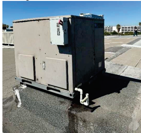
M6 – typical existing rooftop heat pump
