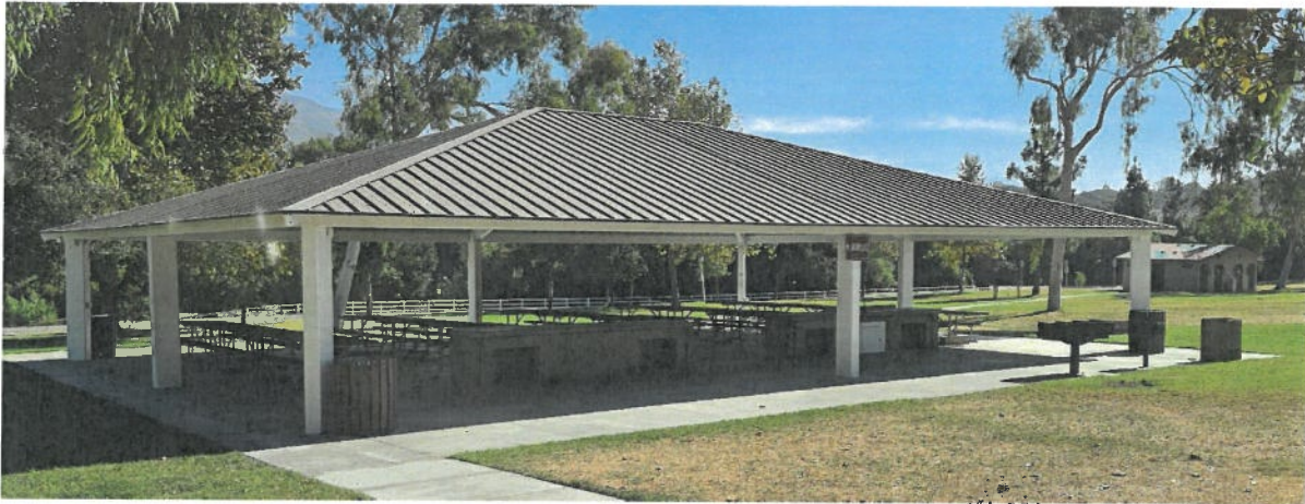
Figure 10 Meadowlark Shelter (Photo provided by Bergman Development Services)
