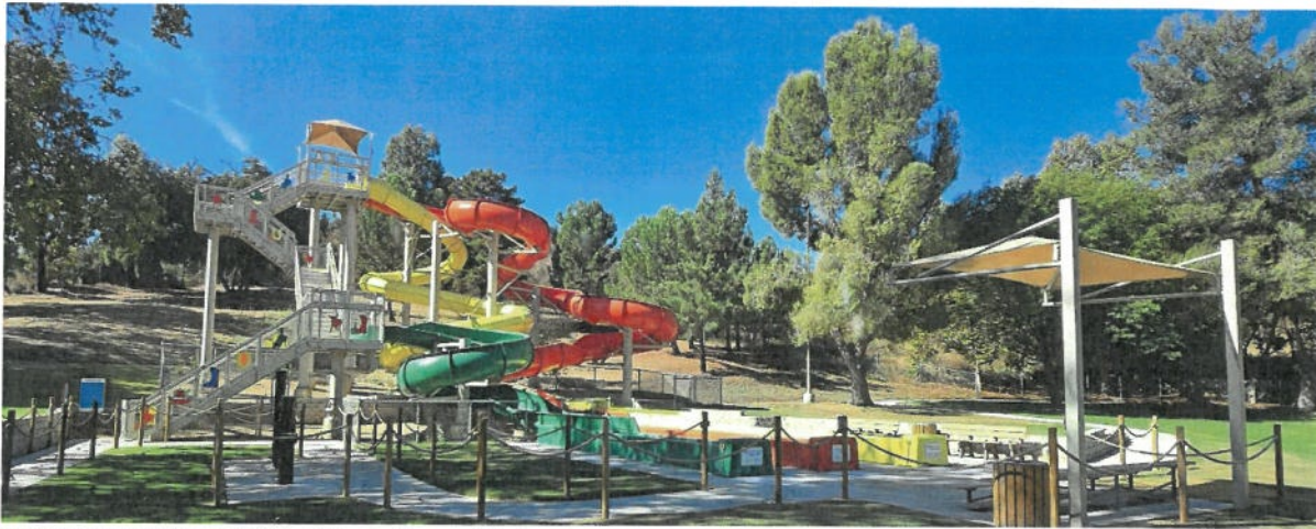
Figure 5 New 3 flume Waterslide and tower (Photo provided by Bergman Development Services)
