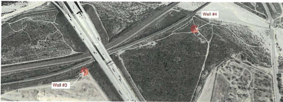
Figure 26 Wells #3 and #4 locations Commissioned by Bergman Development Services
