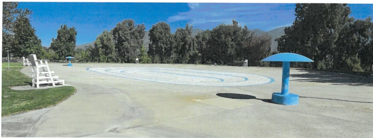
Figure 7 Existing swim basin (Photo provided by Bergman Development Services)
