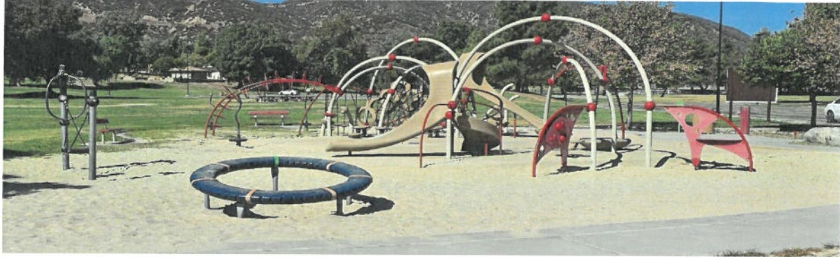
Figure 15 New playground (Photo provided by Bergman)
