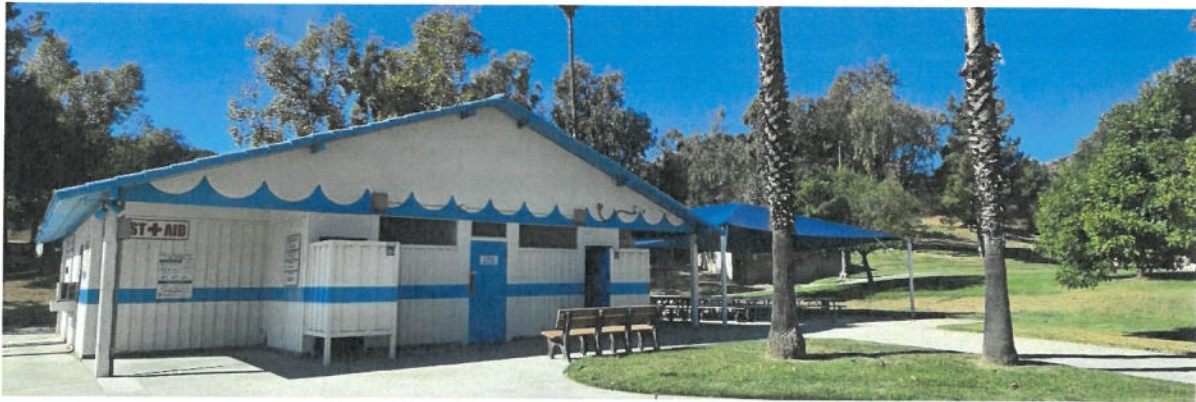
Figure 8 Existing food service, restroom office building (Photo provided by Bergman Development Services)
