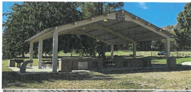
Figure 11 Coyote Shelter (Photo provided by Bergman Development Services)
