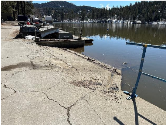
Existing boat launch ramp
