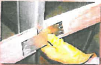
Overlap adjacent pieces when going into the horizontal.
