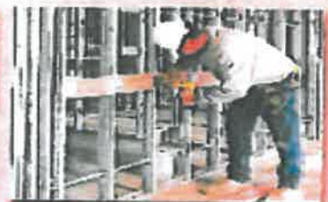
Secure each plate to the steel flange using a small screw or NPS head screw.
