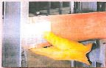
Pop "Starter Edge" into the top side of the stud baffle.
