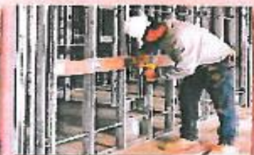
Secure each plate to the stud baffle using a small #8 or #10 self-tapping screw.
