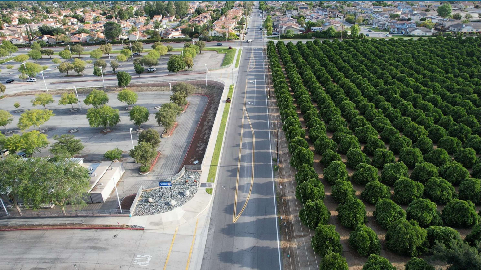
Colton Avenue adjacent to REVHS athletic facilities and parking areas, illustrating multi-lane roadway conditions, student crossing activity, and exposure to vehicle traffic along a key school access corridor.
