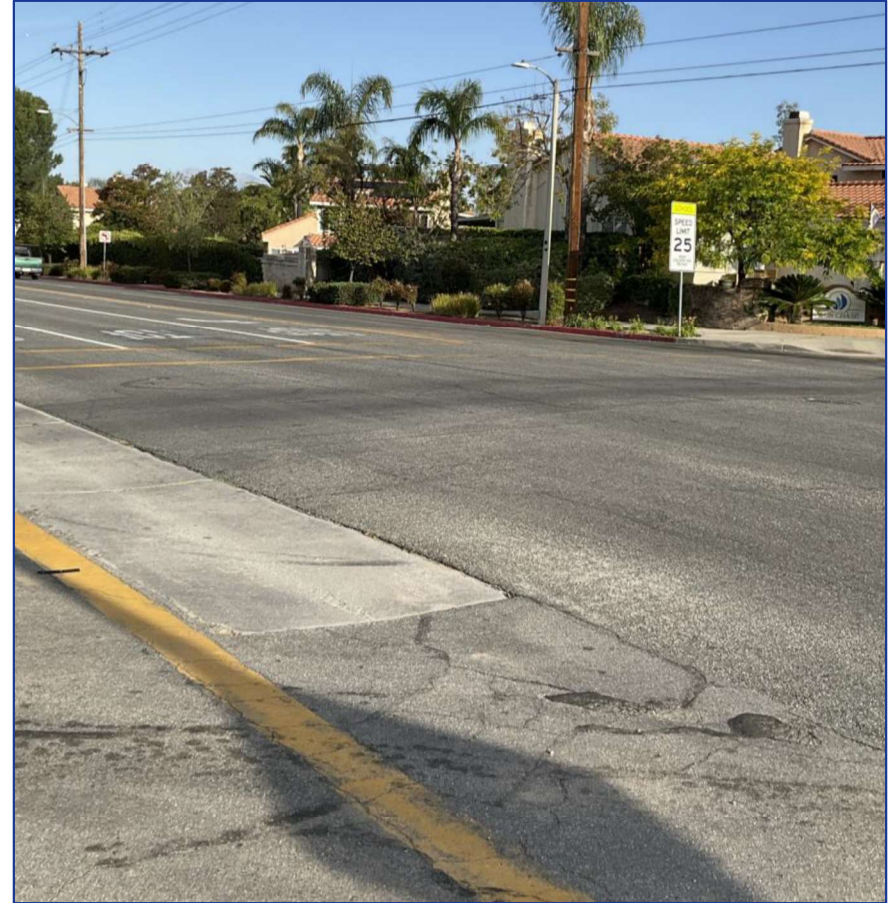
Intersection near Agate Avenue along the Colton Avenue corridor, illustrating wide crossing distances, limited crossing visibility, and exposure to turning vehicles at a key student crossing location.
