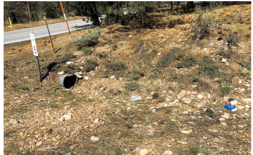
Drainage Two Facing Southwest
