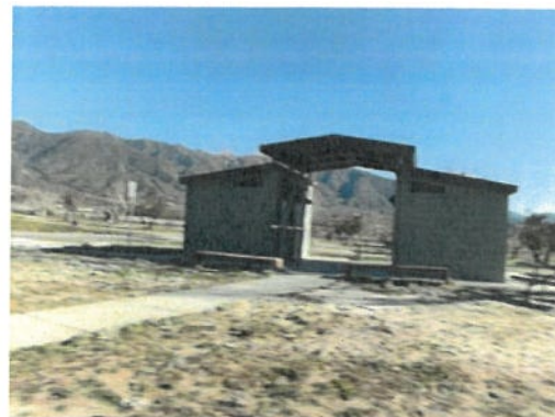
Restrooms for campground
