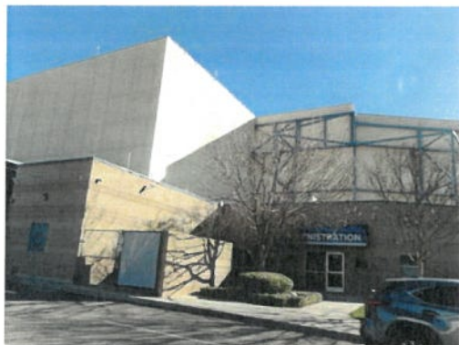
Amphitheater building and offices
