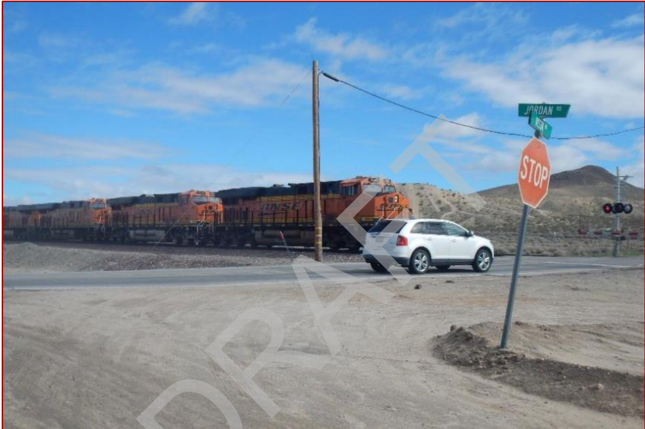
Figure 1. Current At-Grade Crossing: Vista Road at Jordan Road (Facing East)
