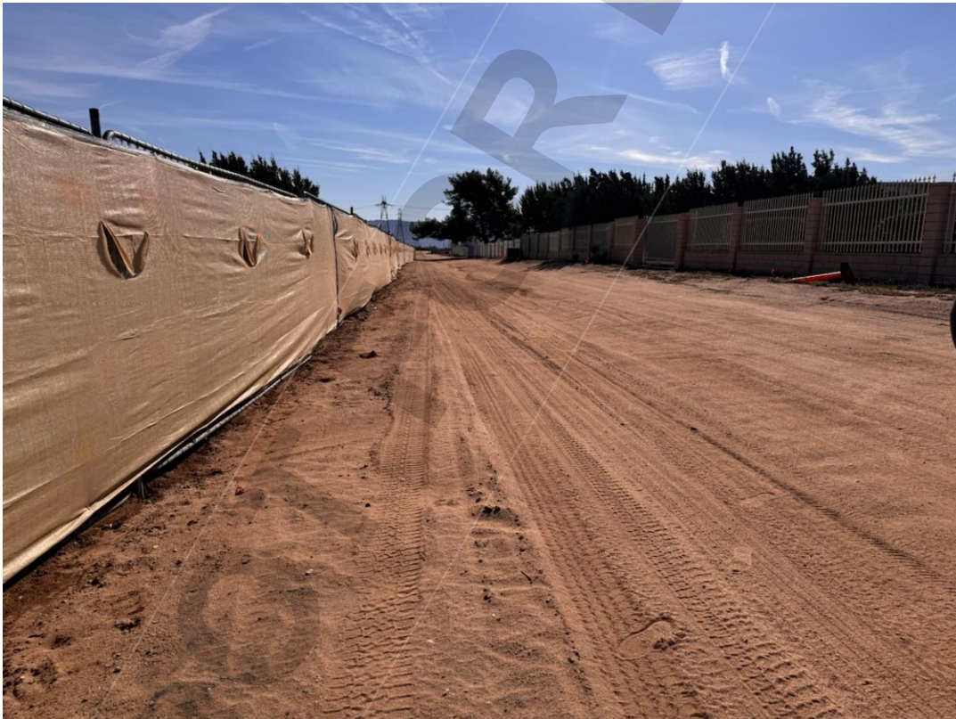
Photograph No. 1, Current alignment conditions at BH-01 on Rodeo Road, view to east.
