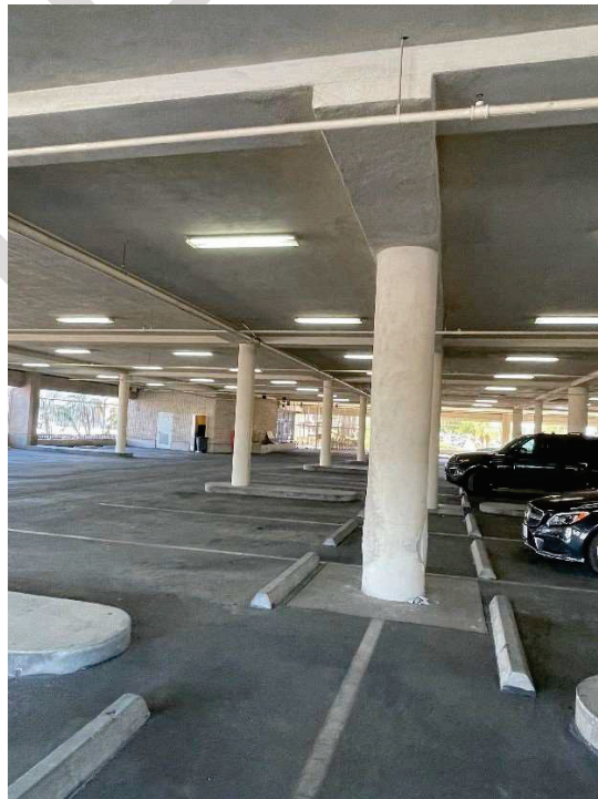
Photo S2 – View of two columns added in previous retrofit
