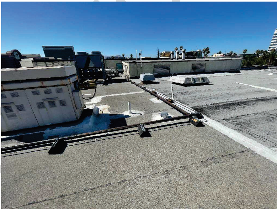
Photo S4 - View of main gas line with no seismic bracing support
