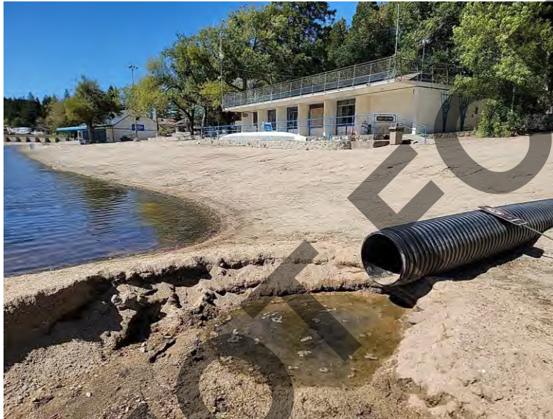
Photograph 5: View facing northwest towards Inlet-13 depicting typical conditions observed at inlets throughout the site.
