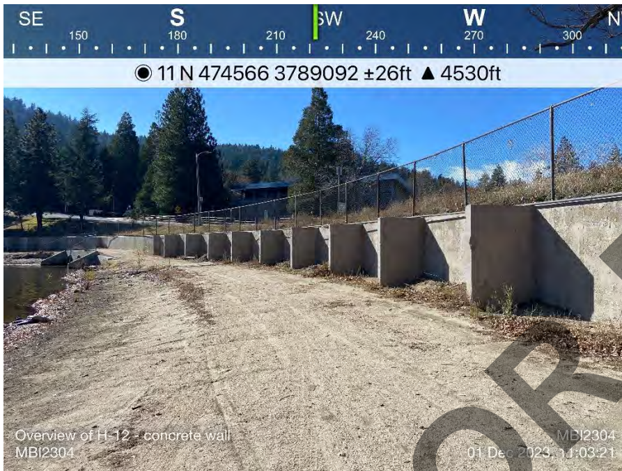
Photo 5: Retainer Wall Overview (View SW)
