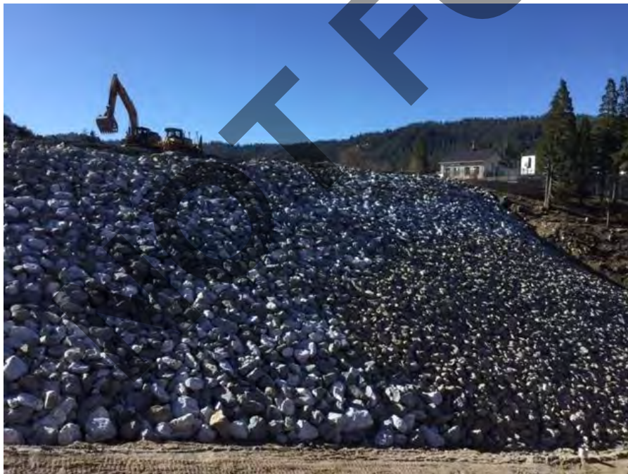
Photo 6: Dam Overview (View NE) Source: San Bernardino County (2019).
