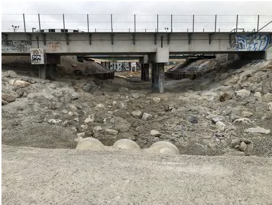
Photo 4: North-facing view of the railroad bridge over the channel.
