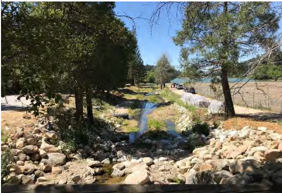
Figure 4 San Moritz Channel/Debris Basin
