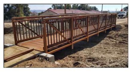
Pedestrian Bridge: H - Section, Pratt Truss Weathering Steel Bridge Railing System: Horizontal angle safety rails with < 4" openings up to a minimum 42" high with toe plate, rub rail, & pipe handrail.
