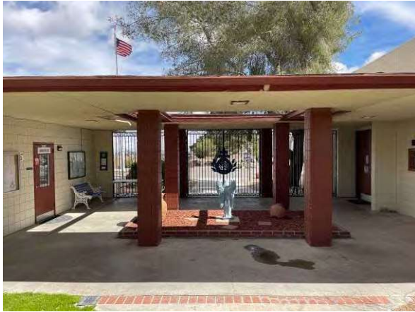
Photo #1 View of front gate to complex, facing north.
