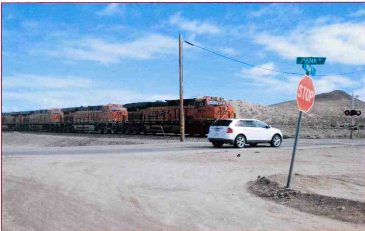
Figure 6-3: Current At-Grade Crossing: Intersection of Vista Road and Jordan Road (Facing East)
