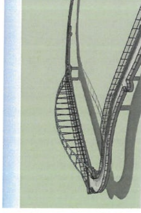
Prefabricated bridge capable of well over 100'
