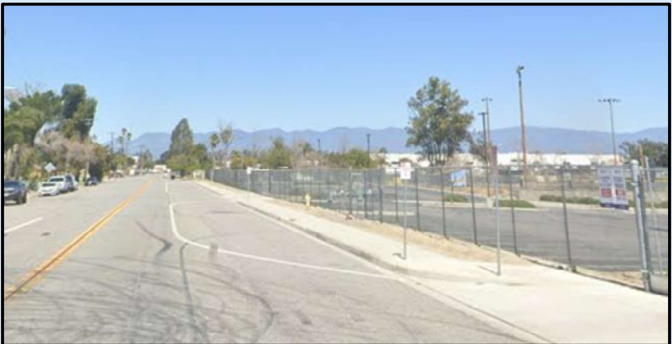
Photo 10. Intersection of Laurel Avenue and Avenda Cortez facing north. Lack of ADA-Accessible ramps. Students frequently cross this intersection. The project will include a high-visibility crosswalk with push-button control rapid flashing beacons at this location.
