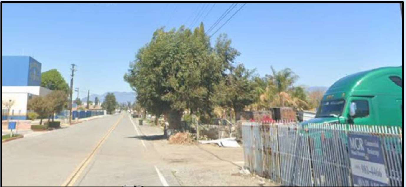
Photo 2. Laurel Avenue facing north directly across from Bloomington HS. Lack of sidewalks and obstructions limit pedestrian use. An unmark dirt driveway to a business utilizing semi trucks creates additional safety concerns for students and residents traveling from the eastern neighborhoods.
