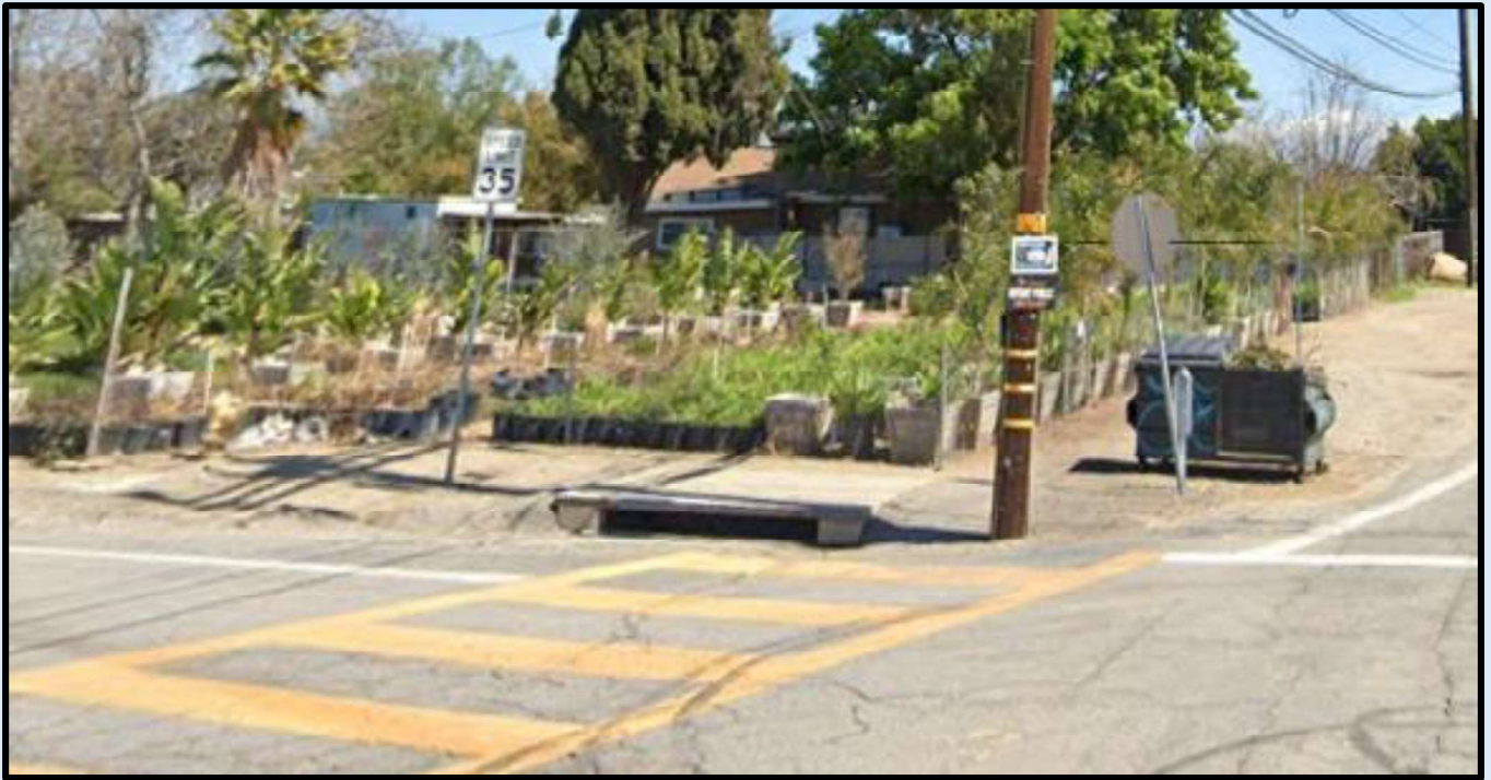
Photo 9. Intersection of Laurel Avenue and Santa Ana Avenue facing east. Lack of sidewalks, curb and gutters, and ADA-Accessible ramps. The proposed project includes sidewalks, ramps, and curb and gutter at the three missing corners (northeast, southeast, and southwest) and sidewalks along the east side of Laurel Avenue and the north and south sides of Santa Ana Avenue.
