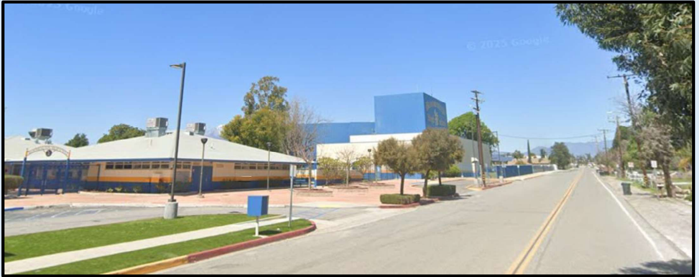
Photo 5. Laurel Avenue facing northwest. Students frequently cross midblock in front of the school during pick-up and drop-off times with heavy traffic. The project will install a high-visibility crosswalk with push-button control rapid flashing beacons at this location.
