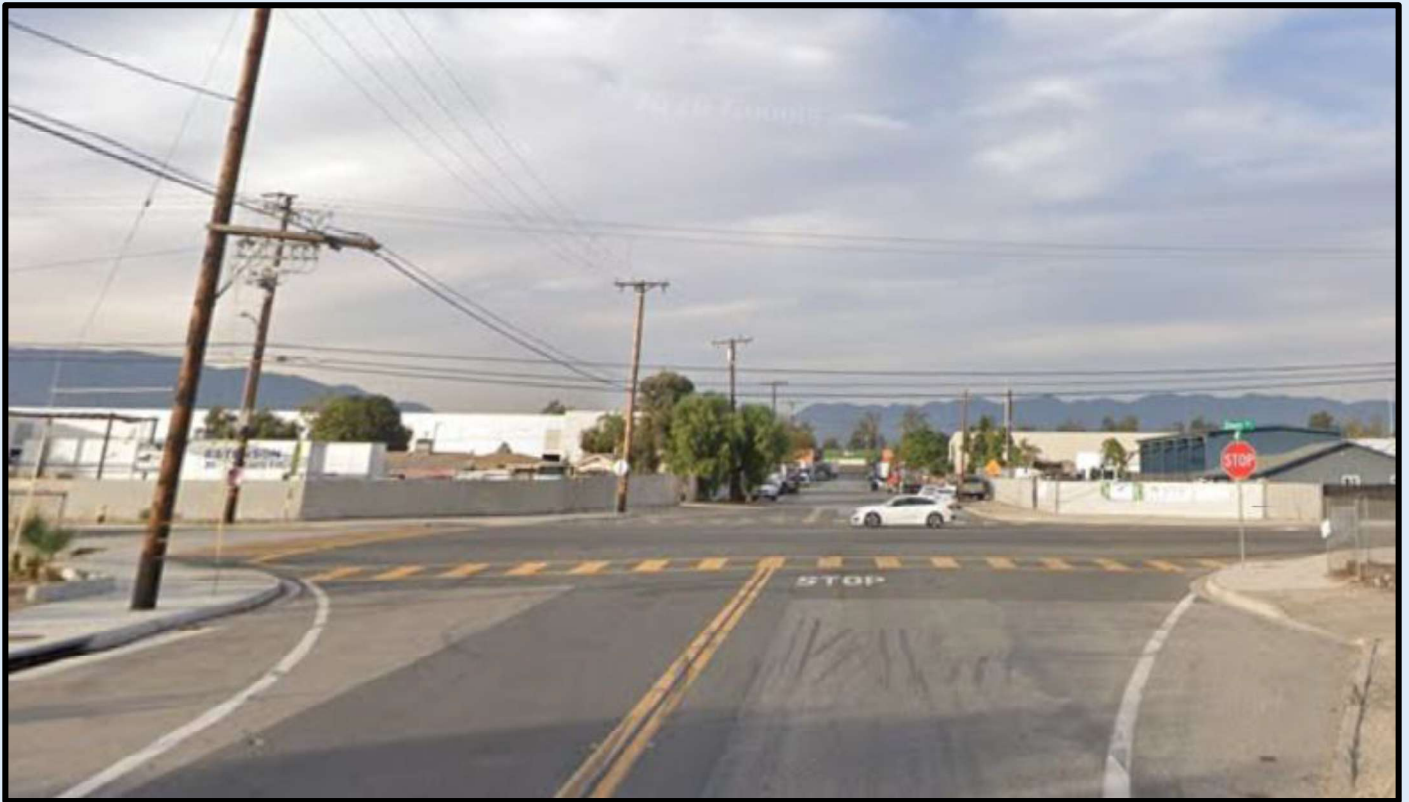
Photo 7. Intersection of Alder Avenue and Slover Avenue facing south. The Project includes a proposed traffic signal to replace the four-way stop at this intersection, which is inadequate for managing the high-volume surges seen during peak times such as school pick-up and drop-off periods.
