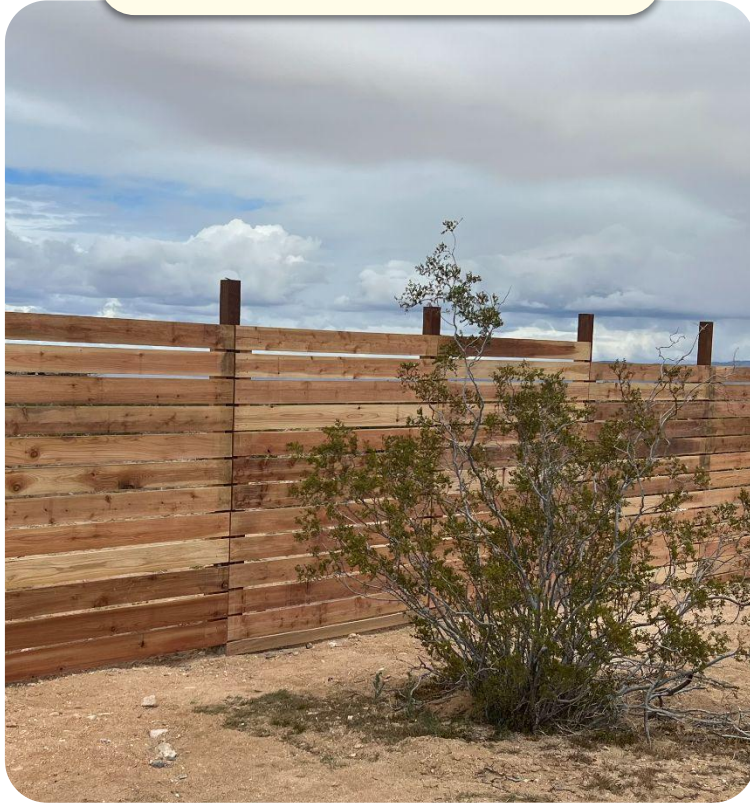
5 foot cedar perimeter fencing
