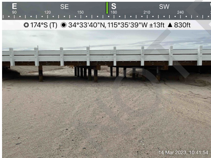
Photo 7: Downstream view of Lanzit Ditch Bridge, facing south on March 14, 2023.
