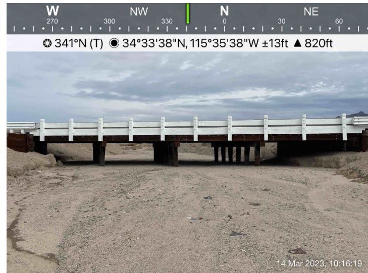
Photo 8: Upstream view of Lanzit Ditch Bridge, facing north on March 14, 2023.
