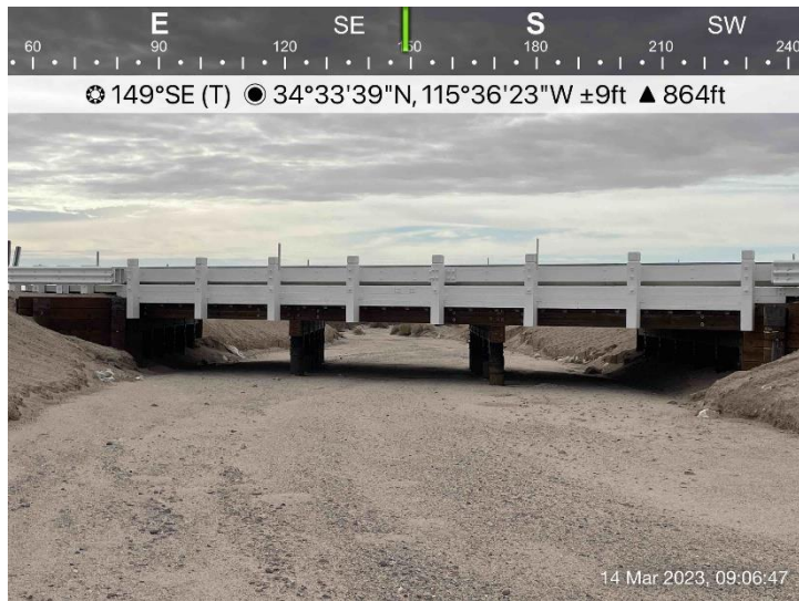
Photo 1: Downstream view of Dolan Ditch Bridge, facing south on March 14, 2023.
