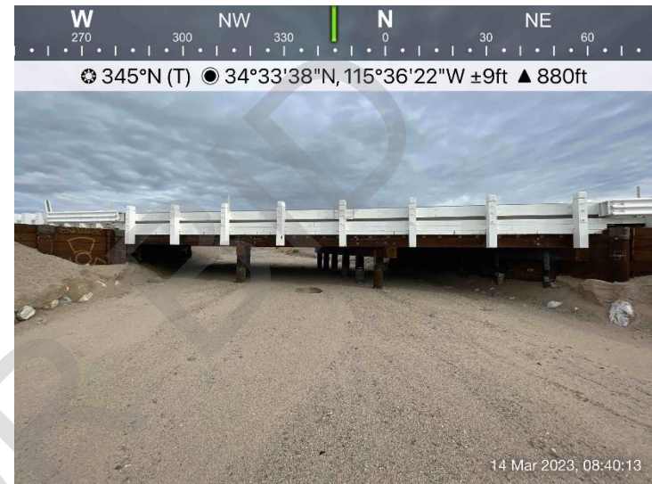
Photo 2: Upstream view of Dolan Ditch Bridge, facing north on March 14, 2023.
