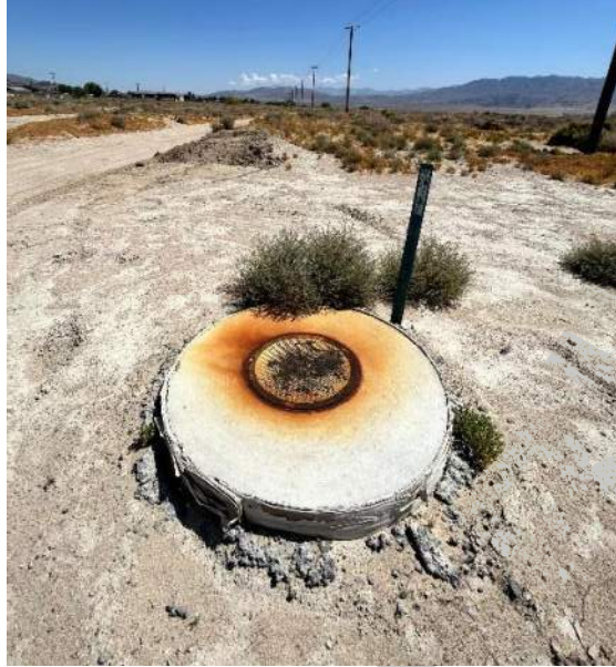
Figure 2-3 Sewer Manhole and Cover Replaced in 2019
