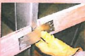
Overlap connector plates when coming into a turning angle.
