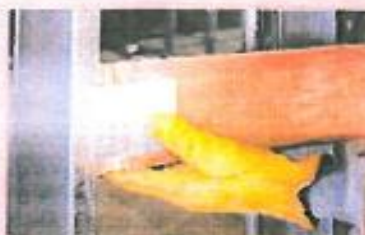
Step 1: Insert "Starter Edge" into the up side of the stud flange.
