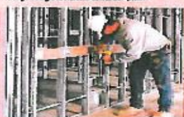
Secure each plate to the stud flange using a small 3/8" or 1/2" head screw.
