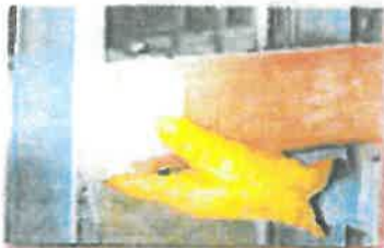
Step 1: "DABACK" backing sheet is inserted into the space between the studs.
