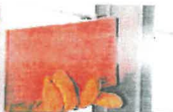
Step 2: "DABACK" backing sheet is inserted into the space between the joists.
