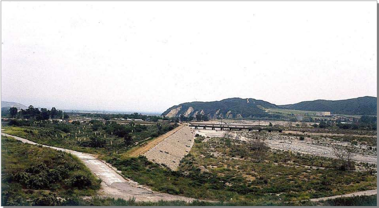
Flood control facilities within the site (circa 2005)
