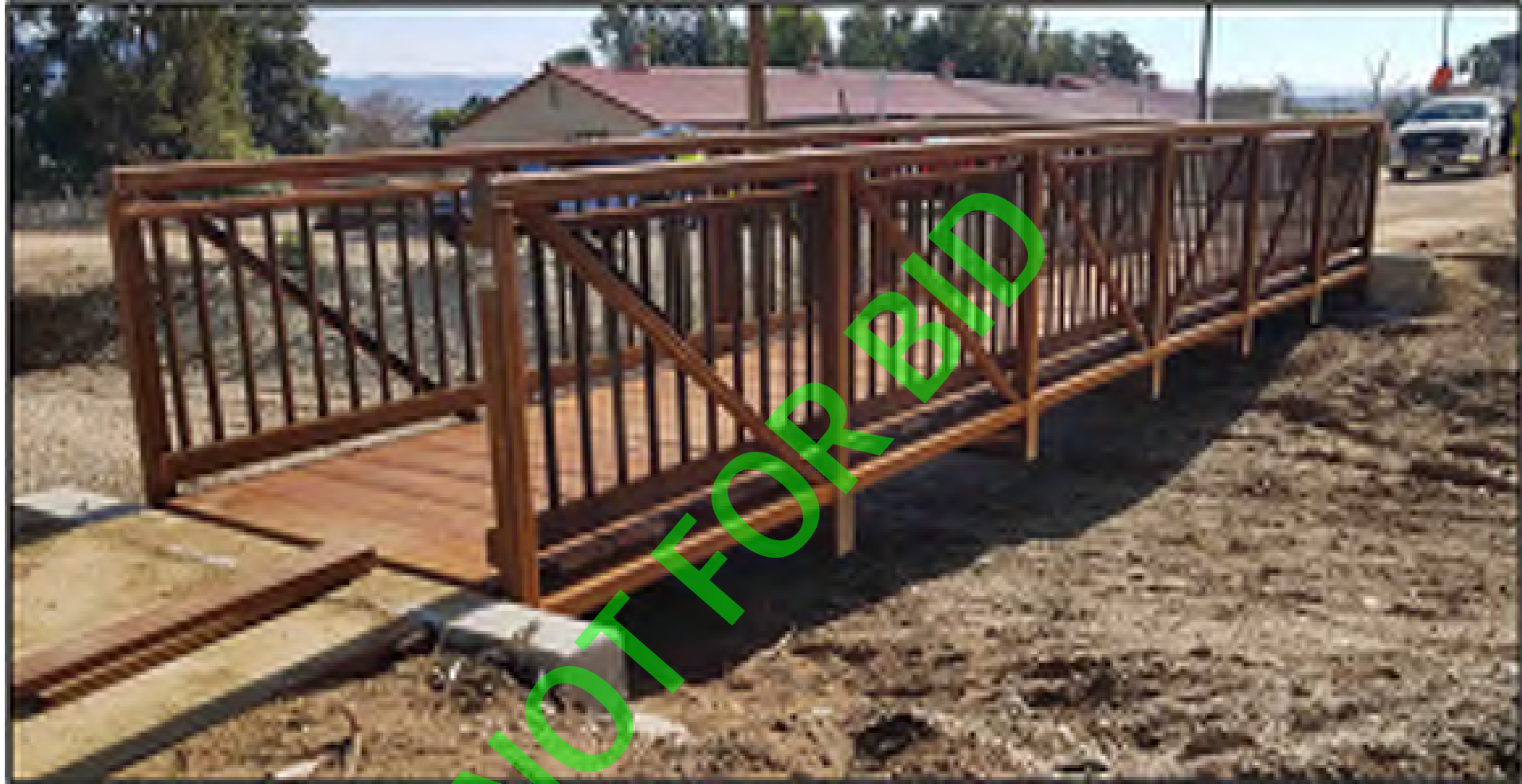
Pedestrian Bridge: H - Section, Pratt Truss Weathering Steel Bridge Railing System: Horizontal angle safety rails with < 4" openings up to a minimum 42" high with toe plate, rub rail, & pipe handrail.
