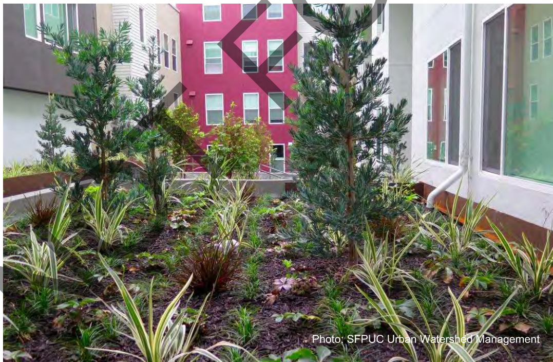
Figure 3. Downspout to mulched flow-through planter bed in project courtyard.
