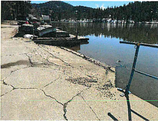
Existing boat launch ramp
