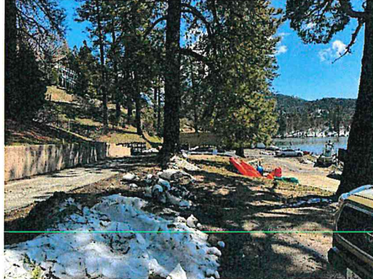
Existing access roadway and parking
