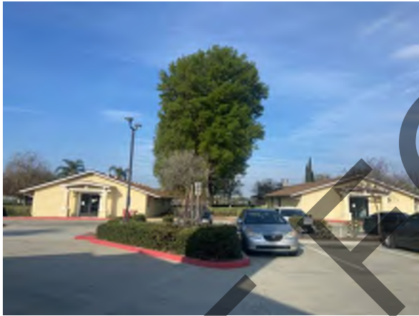
Photo #9 View of the office building and kitchen on the western portion of the site.
