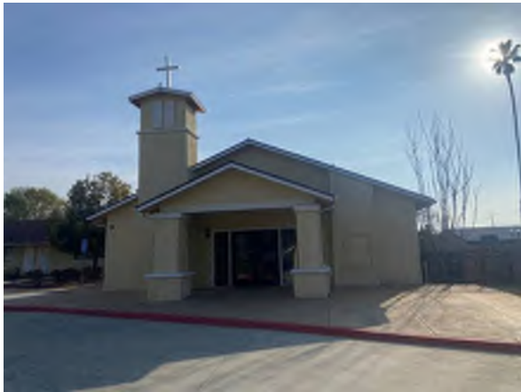
Photo #7 Typical view of the chapel located on the central portion of the site.
