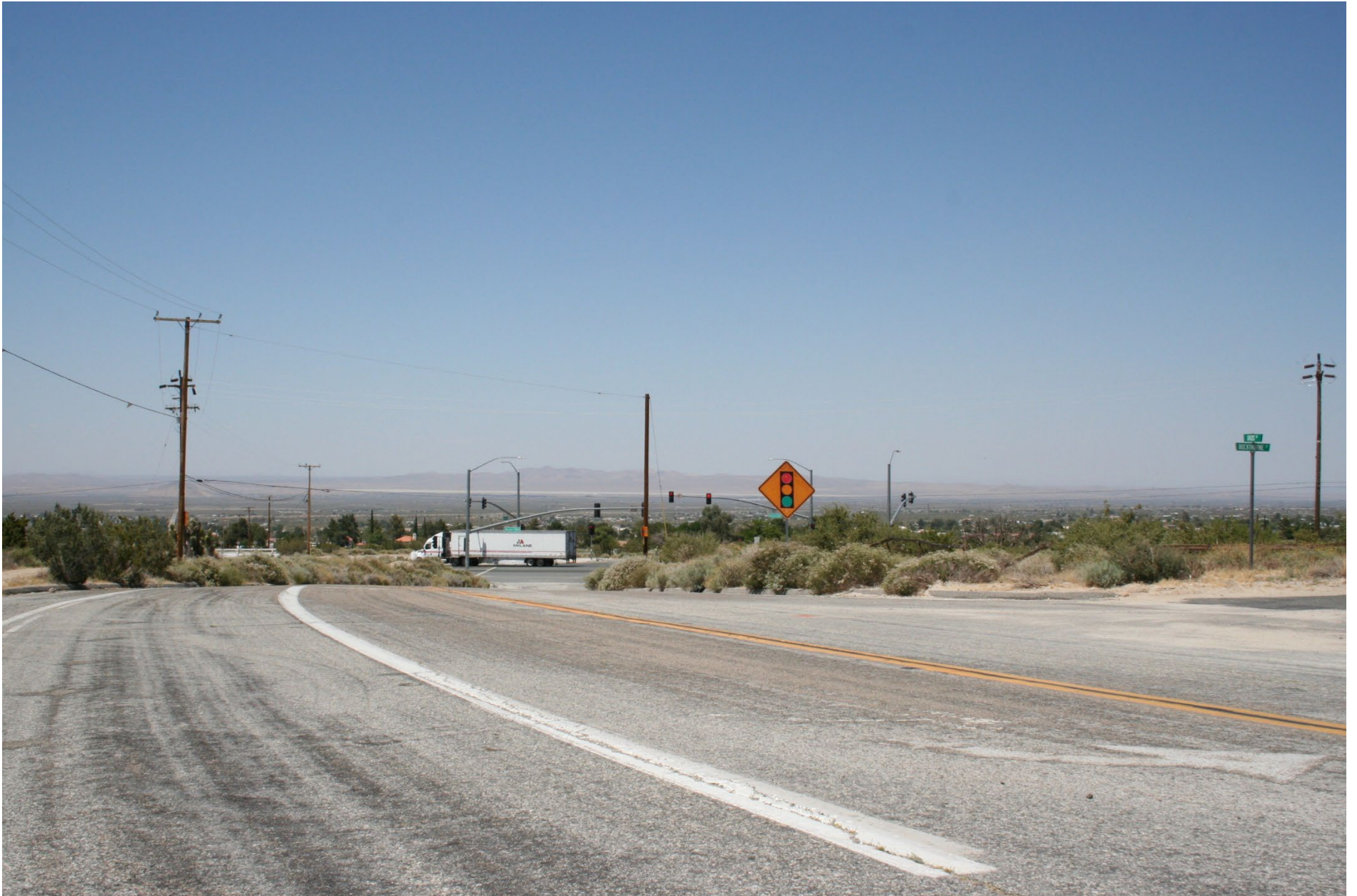
Limited sight distance at Post Office driveway
