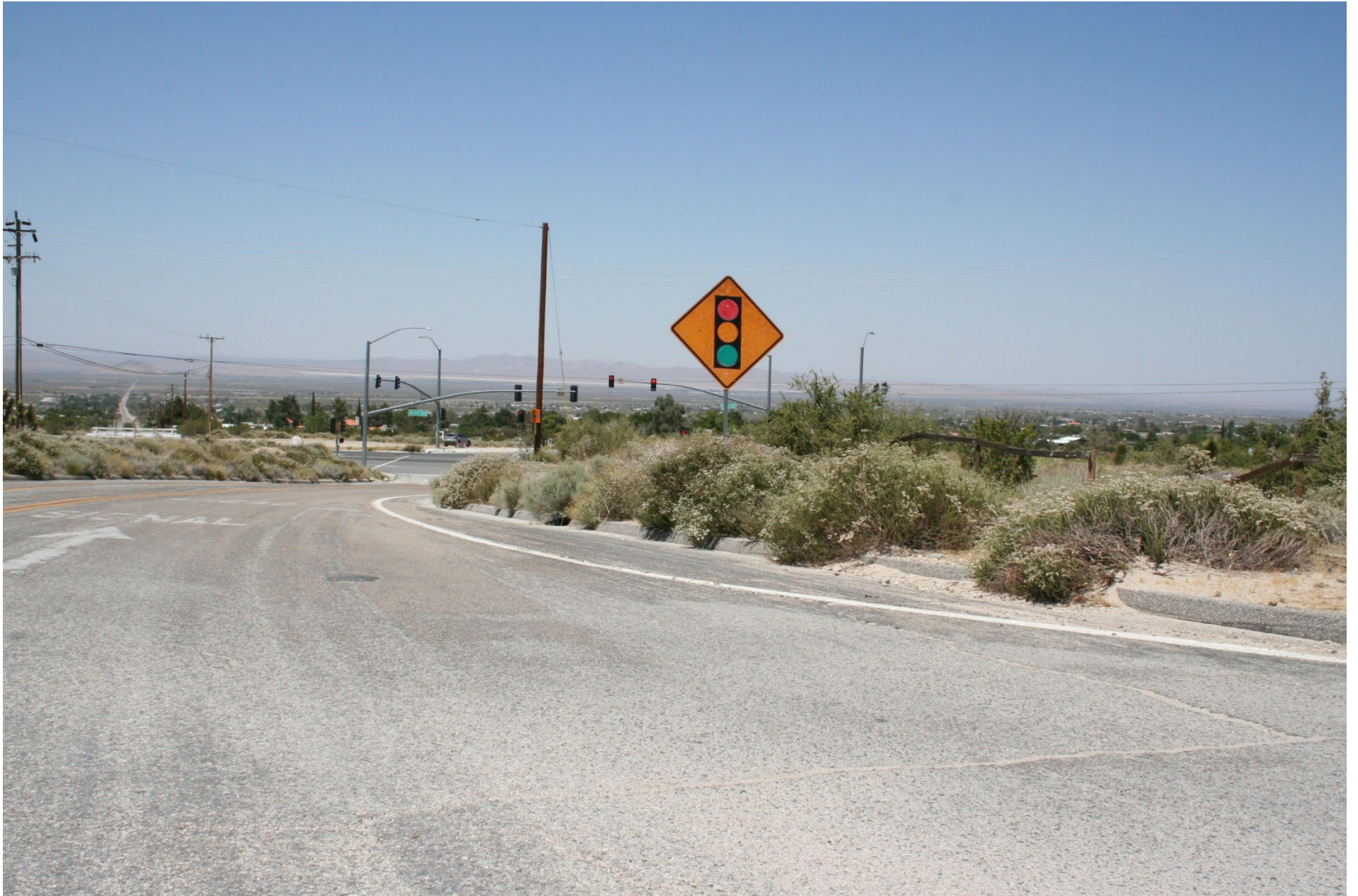
Limited sight distance at Buckthorne Rd
