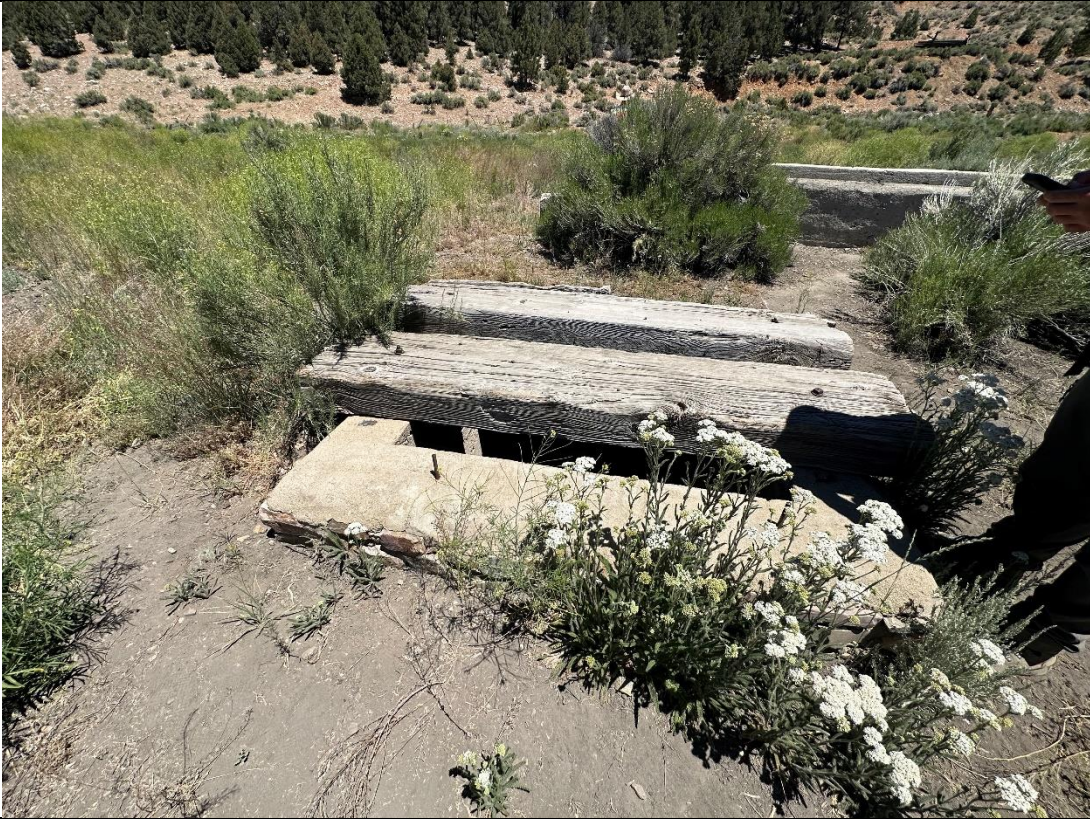
Photograph: 3 Abandoned mine shaft located on the northeast side of the Subject Property.
