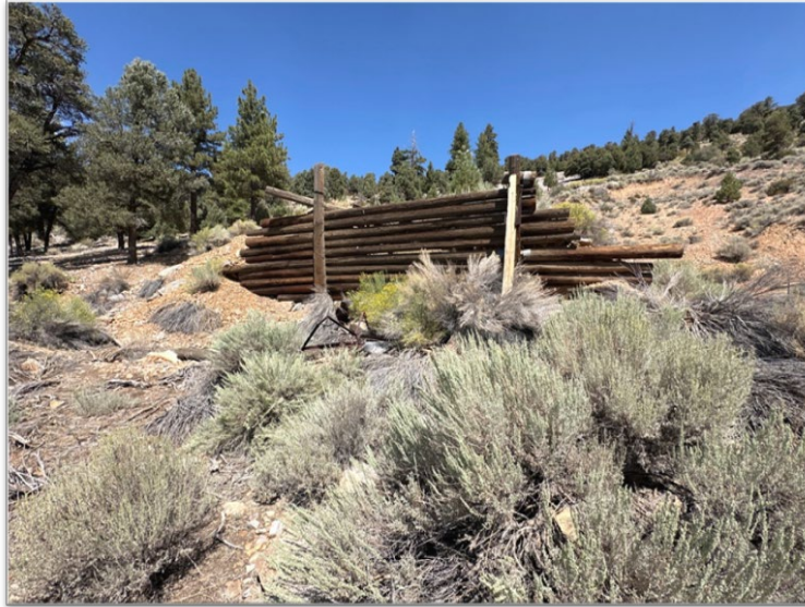
Photo 25. Overview of Locus 3 with Feat-6 (mine adit) and Feat-7 (remains of mining equipment). View towards north.
