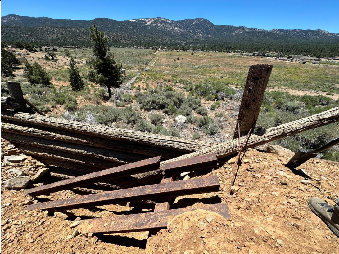
Photograph: 5 | Production shaft that has been backfilled with soil and covered with a metal grate located on the northeast side of the Subject Property.
