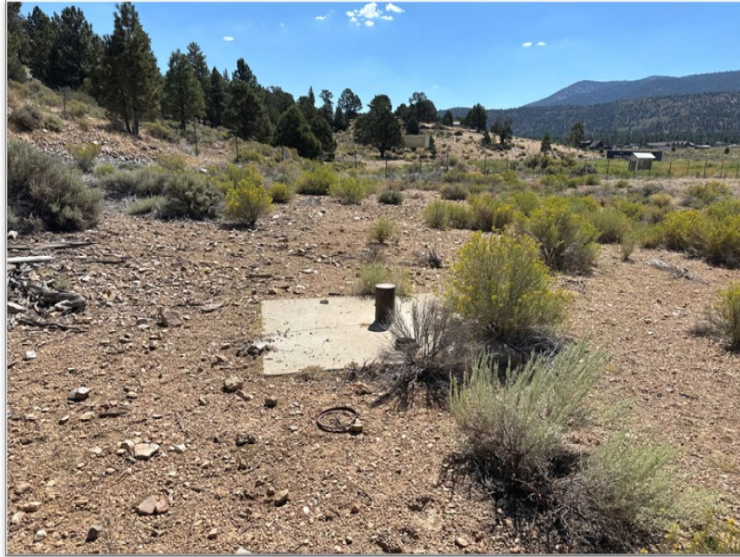
Photo 15. Feat-4 consisting of ventilation shaft. View towards east.
