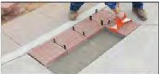
Step #3 - Thin Set Installation - Set pavers. Be sure pavers are fully set into thinset. (Back buttering may be necessary).
