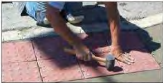
Step #2 - Wet Set Installation - Level pavers by tapping with rubber hammer. Note: Joints may or may not be grouted; contractor option.
