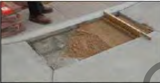
Step #3 - Sand Set Installation - Screed 1/4" masonry sand.
