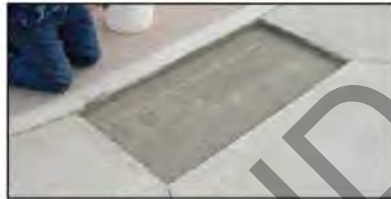
Step #2 - Thin Set Installation - Spread fully and evenly.
