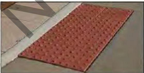
Step #1 - Wet Set Installation - While concrete is still wet, embed pavers into cavity.
