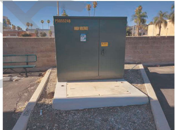
Photo #22 View of the pad-mounted transformer, located on the south-central perimeter of the site.
