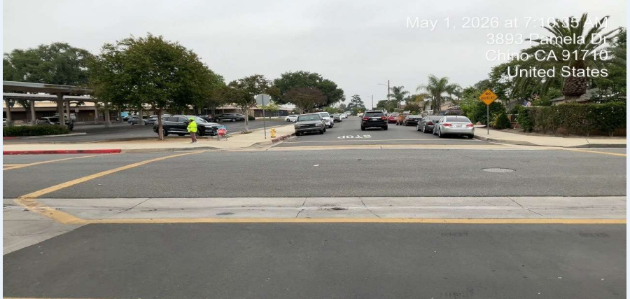
Photo 5. Pamela Dr looking east — vehicles approach the school crossing past a faded painted stop bar.
