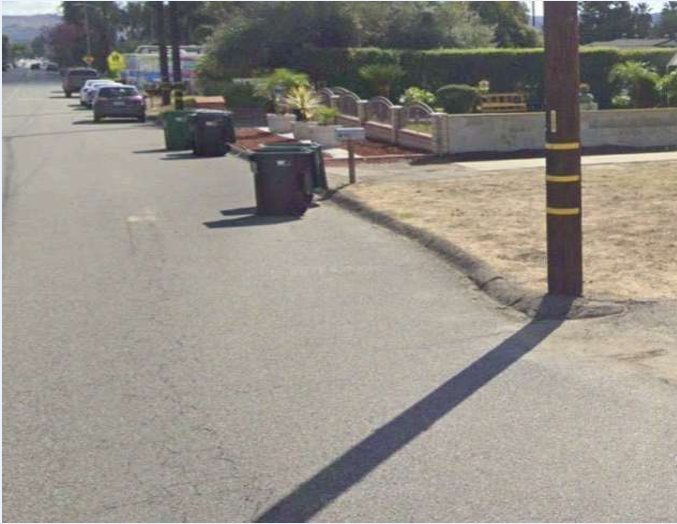
Photo 10. Roswell Ave (Google Street View) — no sidewalk on the west side. Trash cans and pedestrians are forced into the dirt shoulder.
