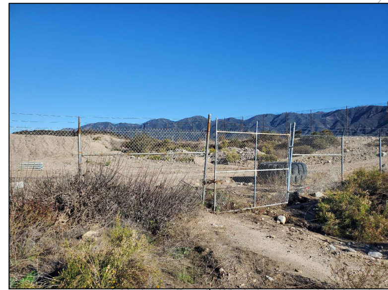
LOCATION #1 OBSERVATION #1: OFFSITE DRAINAGE
