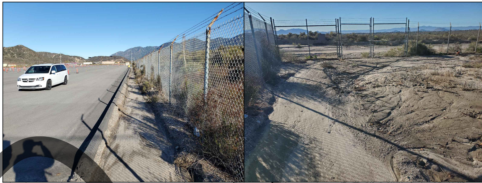
LOCATION #3 OBSERVATION #3: SEDIMENT ACCUMULATES
