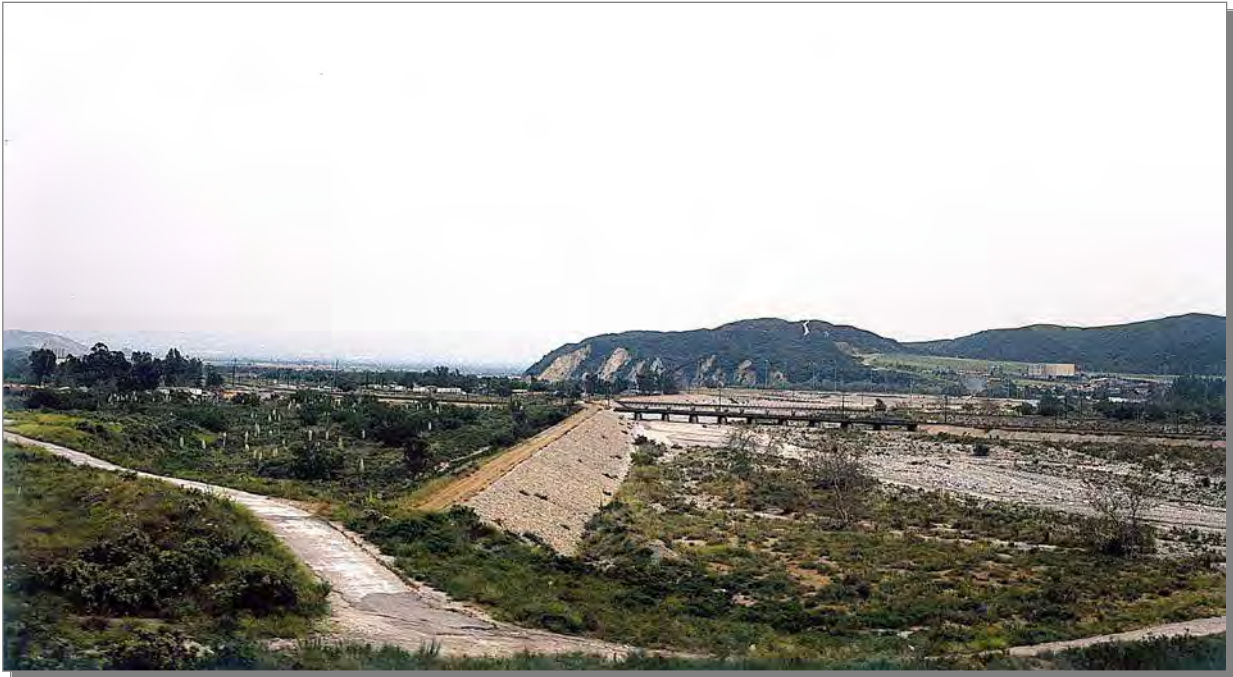
Flood control facilities within the site (circa 2005)
