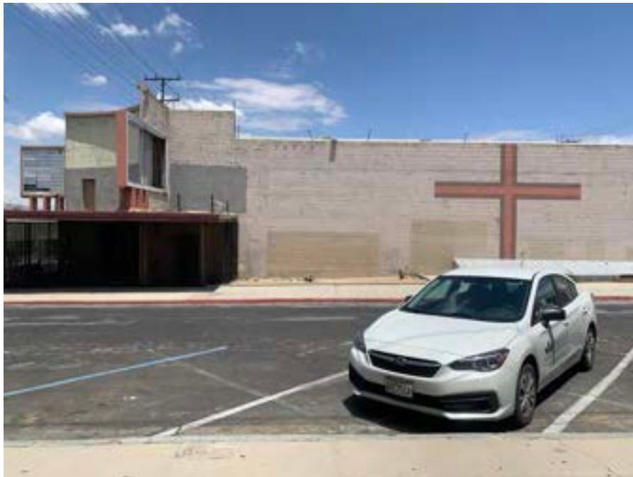
Site Photograph 8 – Looking northeast away from site
