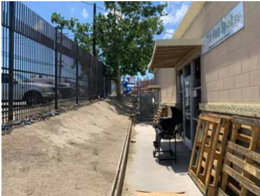
Site Photograph 30 – Playground Walkway
