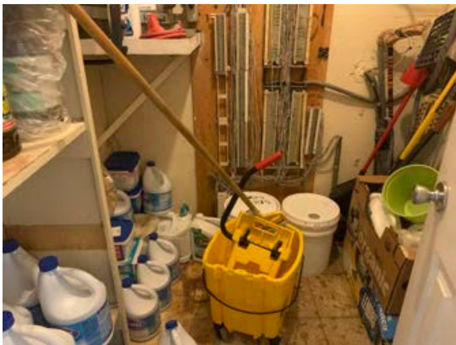
Site Photograph 28 – Interior - Janitor Closet
