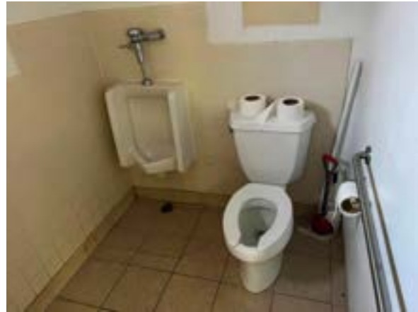
Typical Interior View - Restroom
