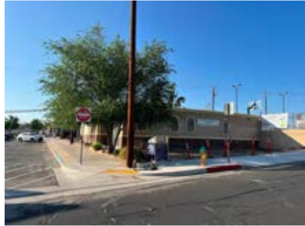
Exterior View – Front/Side
