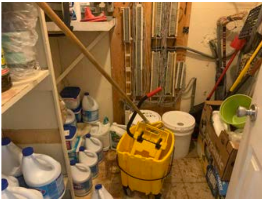
Site Photograph 28 – Interior - Janitor Closet
