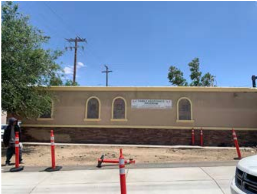
Site Photograph 4 – Looking southeast at site building portion
