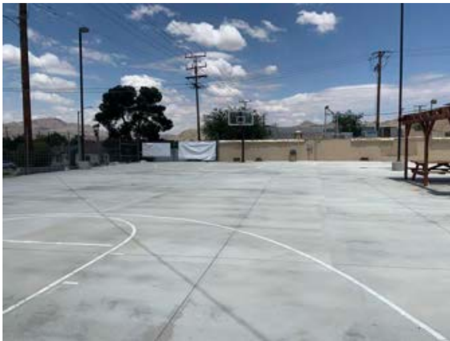
Site Photograph 32 – Fenced Yard - Basketball Court
