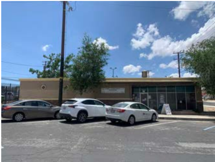
Site Photograph 5 – Looking southwest at site
