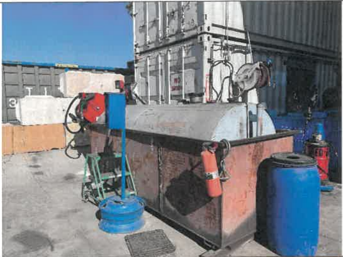
Photo 13. View of 1,000-gallon AST, containing diesel, located outside of the maintenance and storage area. Minor staining pictured.
