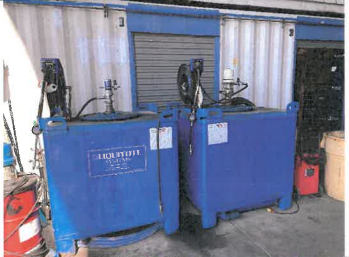
Photo 11. View of two 250-gallon ASTs, containing motor oil and hydraulic oil, located in the maintenance and storage area. Staining pictured.
