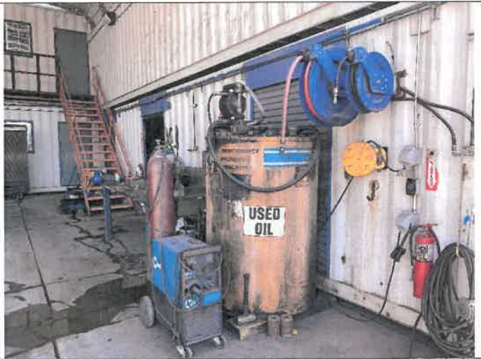
Photo 10. View of 500-gallon aboveground storage tank (AST) containing used oil, located in the maintenance and storage area.
