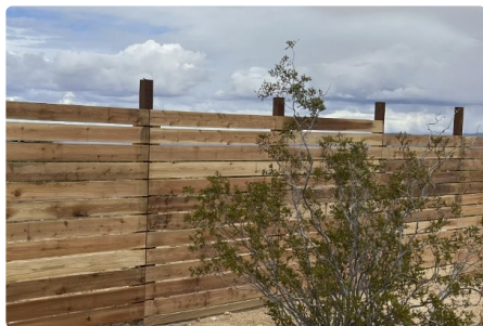
CEDAR PERIMETER FENCING
