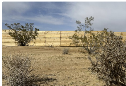
CREOSOTE RETAINED IN PLACE
